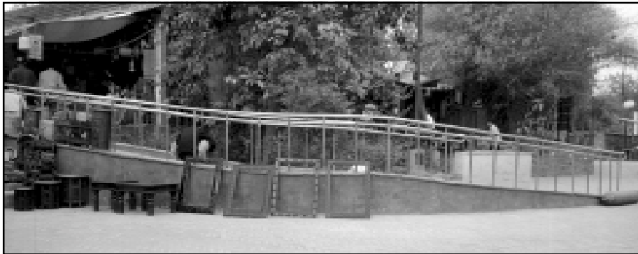
13-metre ramp with landing in Dilli Haat, New Delhi
