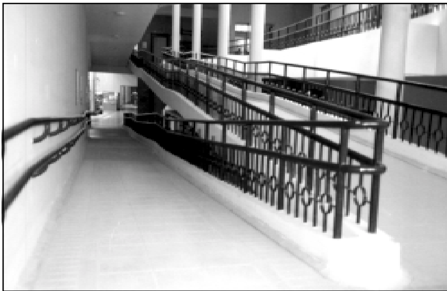
Switchback platform ramp (Photograph: Mobility India, Bangalore)
