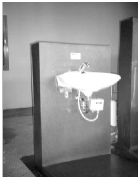
Infra red activated washbasin
