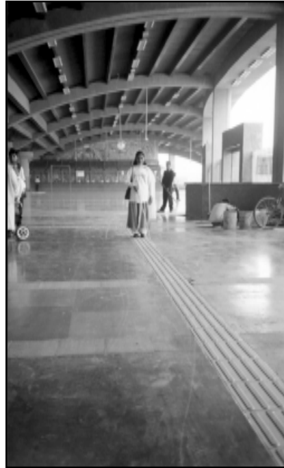
Placement of guiding path and warning strip at the Metro Station.
